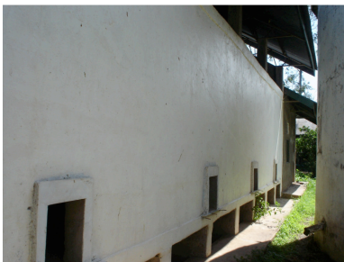
The Namalu silo we will use
