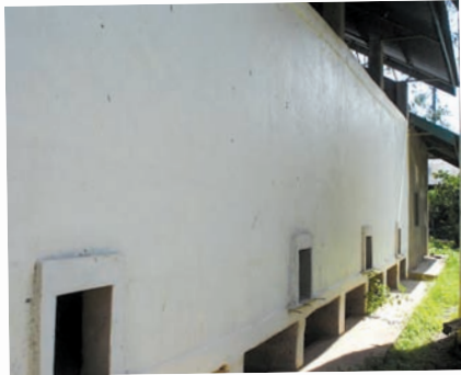
The new food silos at Namalu
